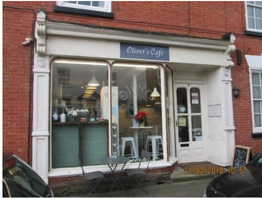
High Street, Kegworth A late nineteenth century shop front
