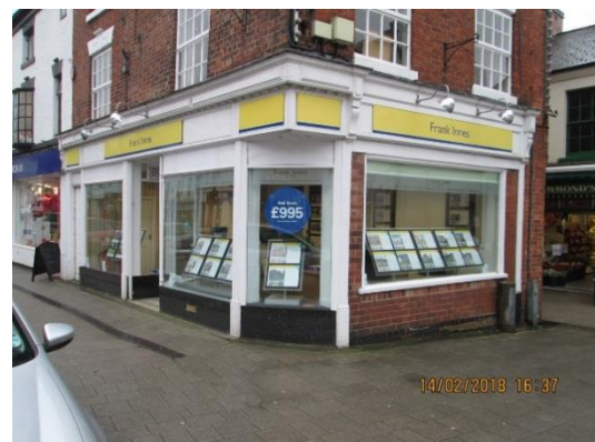
Market Street, Ashby de la Zouch Shop front installed c.1930
